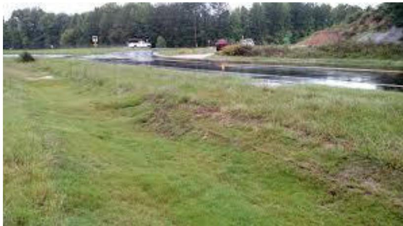
A swale is an elongate vegetated drainage channel designed to capture runoff drainage from upgradient areas of the construction site. The swale is designed to encourage / maximise infiltration of runoff waters through the permeable base / sides as it is transferred to the end point of the swale. The swale is vegetated to provide attenuation of sediment and other pollutants which may be present and therefore also comprises a source-control treatment step.
