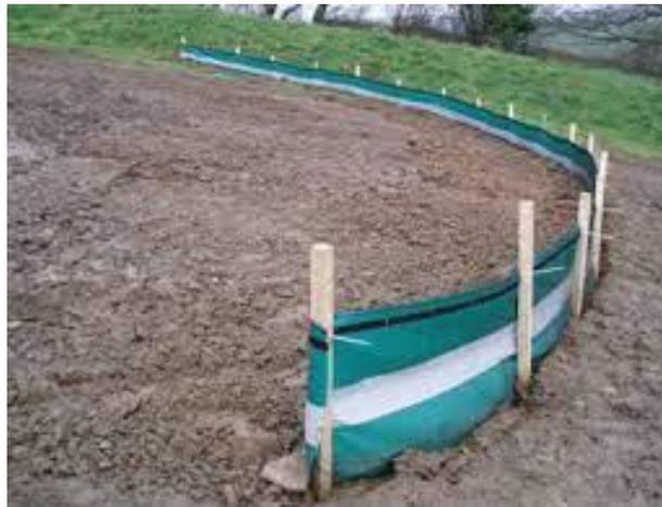
Silt fencing, with associated capture trench, shall be installed across any working areas upflow of the nearest watercourse to act as an emergency capture in the event of failure of other containment measures. Several sections of parallel silt fencing can be installed in high risk situations to act as additional barriers to sediment release.
